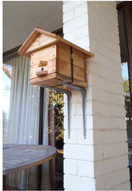
One way to make sure the brackets are level is to put one bracket in first, then line up the 2 nd bracket to make it level.
