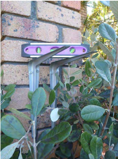
One way to make sure the brackets are level is to put one bracket in first, then line up the 2 nd bracket to make it level.
